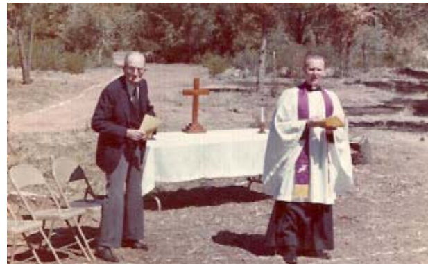
Groundbreaking Service June 1976
